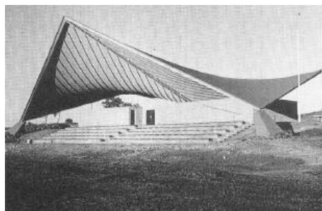
Steel and timber hyperboloid roof grandstand at Mount Newman 1974, Trevor Lewis-Jones with Marie T. Harding ( A pictorial guide to identifying Australian architecture , Apperly et al, p.257).
